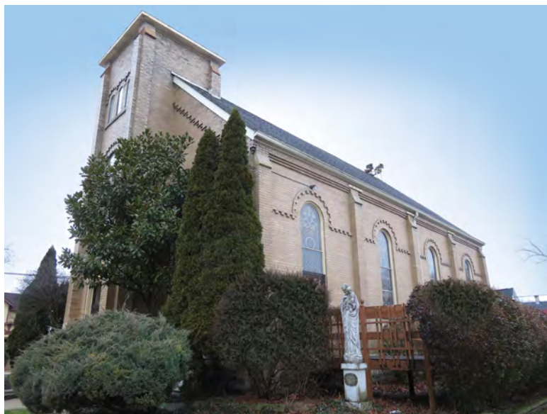
Church: 140 West Avenue
